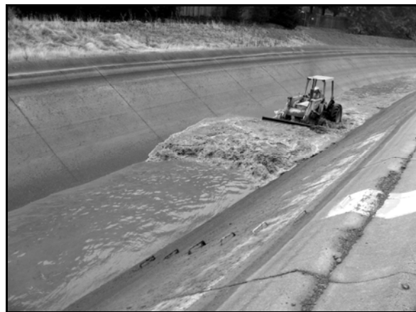
Figure 3. Pushing sediment and vegetative detritus down Union Check at MP 14.80. Photo of November 3, 2006.
