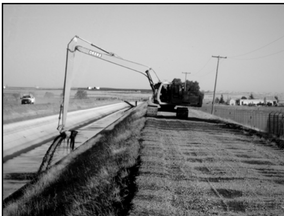
Figure 2. Removal of aquatic weeds and sediment from Sweeney Check at MP 6.15. Photo of October 19, 2006.
