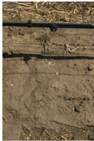
Photo 2. Standard bare berm Note evidence of runoff below drip emitter
